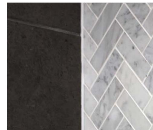
The shower niche and tiled countertop are framed using the **QUADEC** profile in polished chrome anodized aluminum. **DILEX-EKE** creates a smooth wall/floor transition in the shower.
