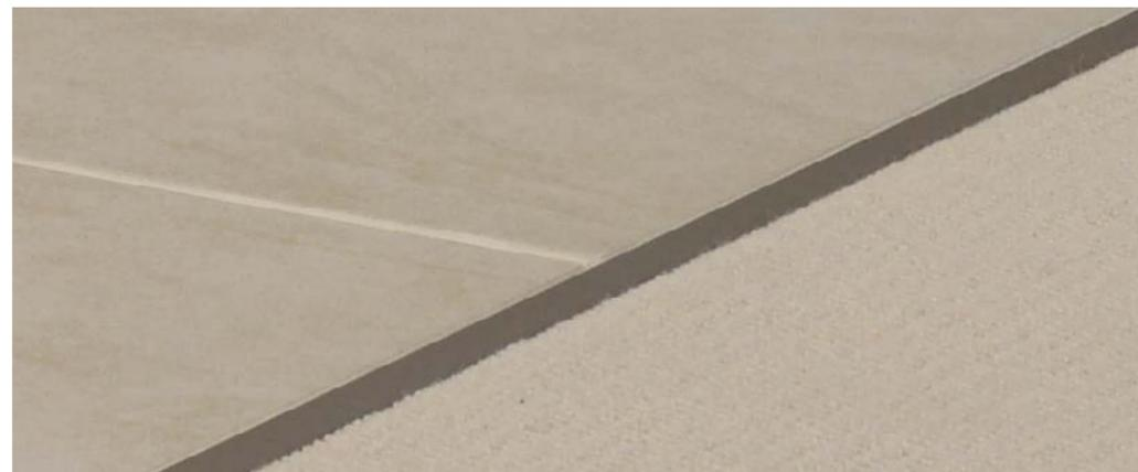
**RENO-TK** floor profile used to create a smooth transition between the tile and carpet. **RONDEC** bullnose profile and matching corners used to finish the edges of the tile base. **DILEX-EKE** PVC corner movement joint profile used to create a seamless transition between the floor and wall.
